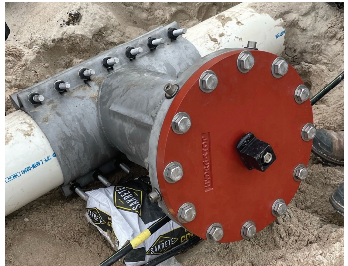
Figure 1. An insertion valve that can be installed at any angle can help facilitate a quick repair in tight confines or difficult-to-access pipes.
