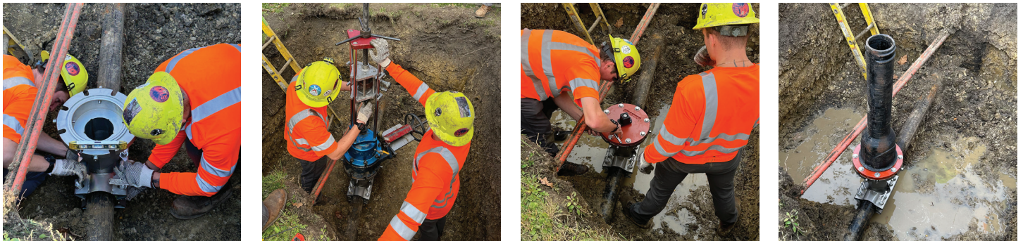
Figure 1. Many valve repair or installation projects can see significant savings by using an insertion valve rather than a traditional valve. A two-man team in the image above was to install a 4" Insta-Valve 250 in Central Illinois in about an hour.
