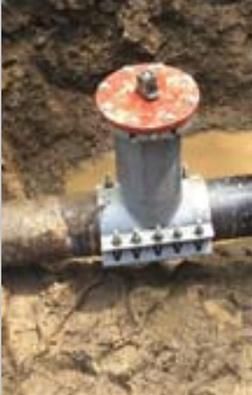
8 inch Insta-Valve 250 Patriot installed on 250 psig transmission line.
